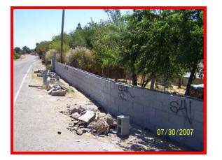
**DO NOT** build fences or walls running parallel to the levee closer than ten feet from the land side toe.
