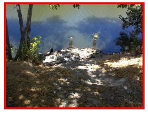
**DO NOT** burn debris on levees, embankments or in channels. The soil bakes, degrading its structural integrity, causing the soil to crumble and be easily washed away.
