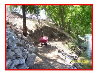
**DO NOT** build steps, retaining walls or any other structure into a levee face.
