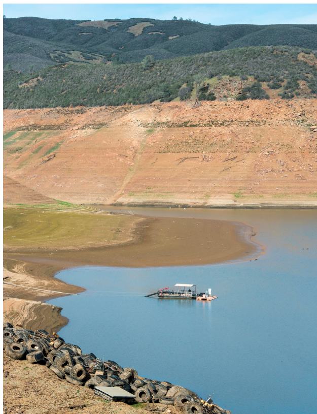
Lake McClure in February 2015, when the reservoir had dropped to only 6 percent of capacity, showing the temporary emergency pumping station (on a barge in the lake) used to divert water to the Lake Don Pedro Community Services District's intake after the intake was stranded by dropping reservoir levels.
