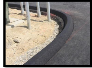
Asphalt Dike at Existing Cushions
