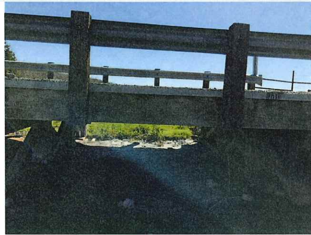
Photo 11 Check in the left exterior girder in Span 1
