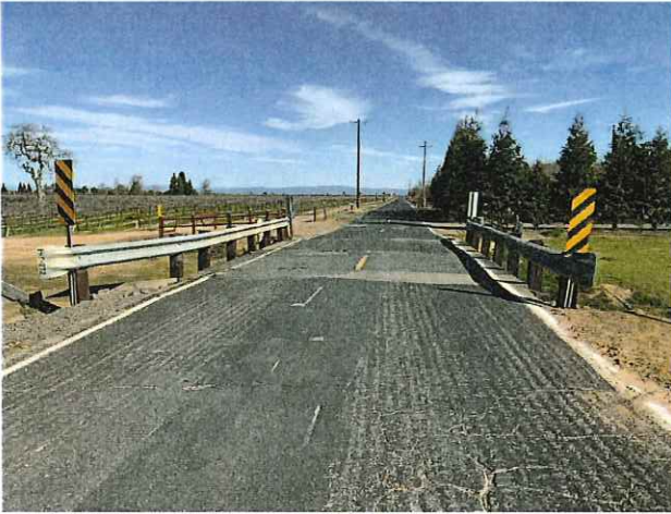
Photo 1 Looking east at Abutment 1
