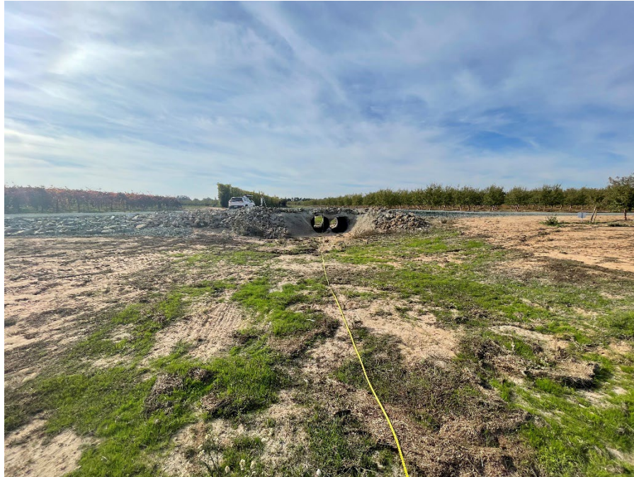
Figure 5. Private Culvert Downstream of BR 29C0272
