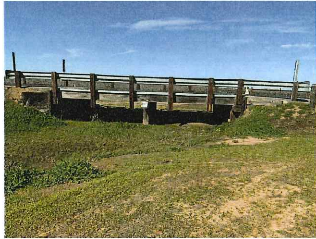
Photo 2 Looking north at the right side of the structure
