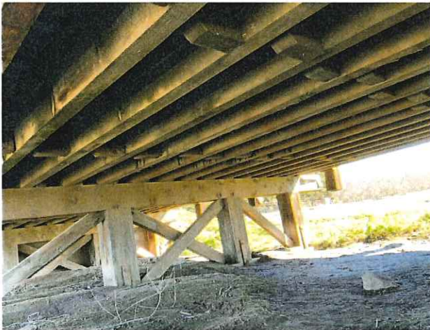
Photo 3 Looking southeast from Abutment 1
