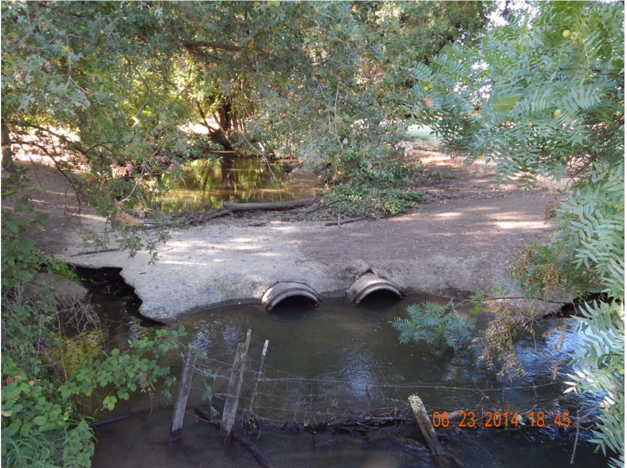
Figure 8. Looking upstream from the bridge. The channel is clear and the overbank areas are vegetated contributing to a higher n -value. Existing low water crossing also shown.
