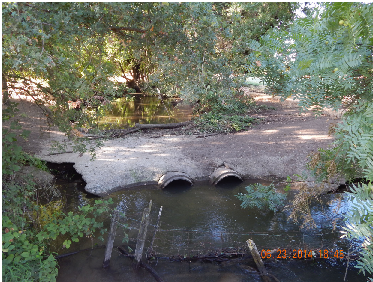
Figure 6. Looking upstream from the bridge. The channel is clear and the overbank areas are vegetated contributing to a higher n-value. Existing low water crossing also shown.
