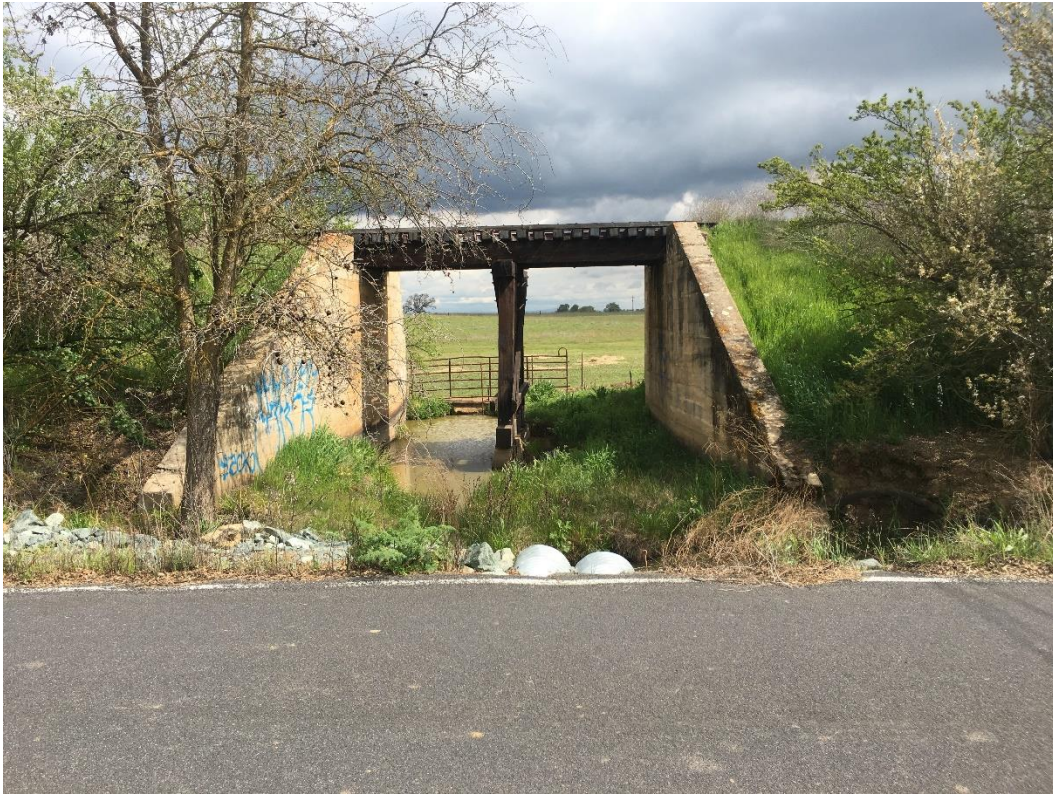
Photograph 3: Middle of Kennefick Road, looking east at the railroad crossing.
