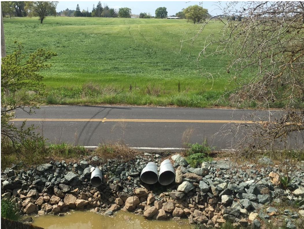
Looking west at the culverts for proposed replacement.
