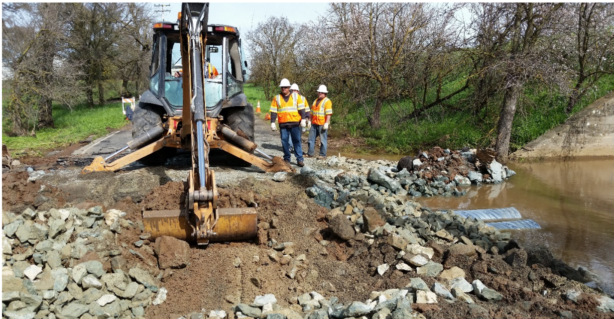
Exhibit 2 – looking east; Railroad bridge wingwall in right side of picture.
