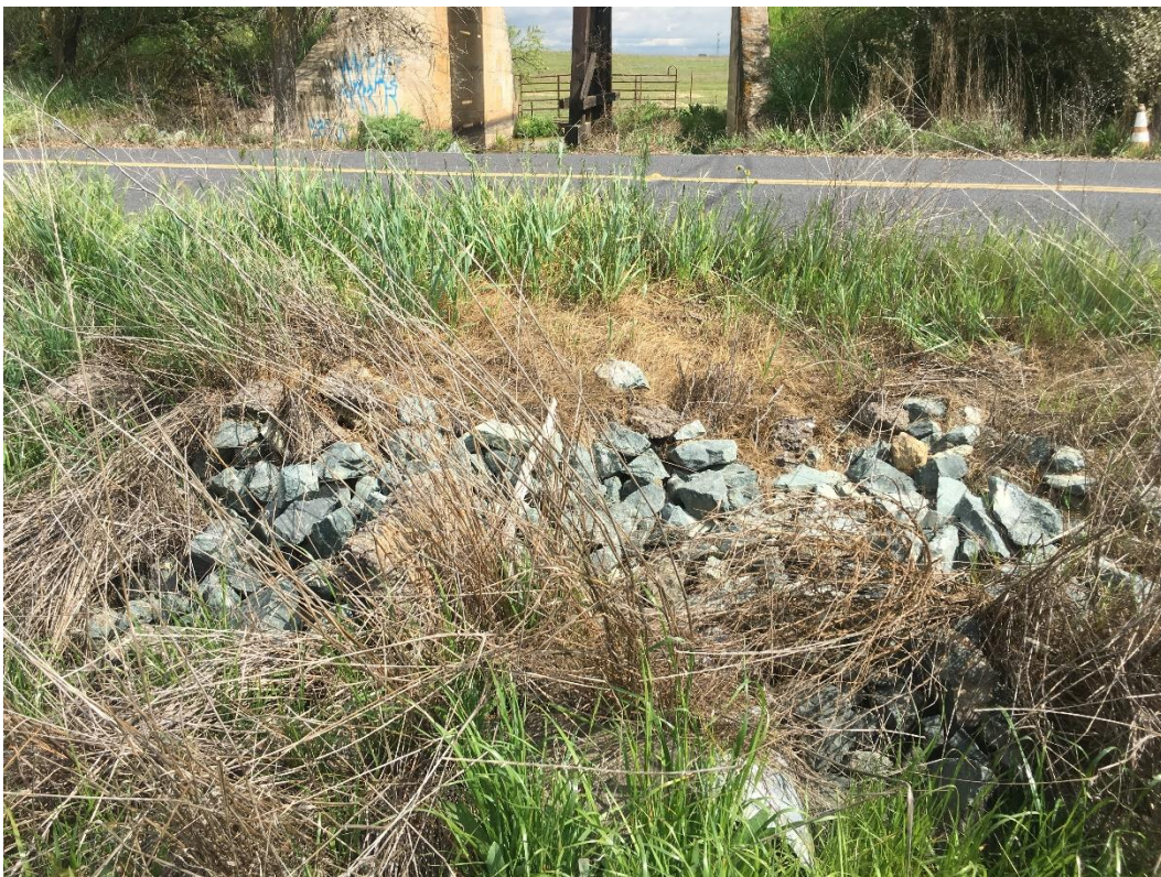
Photograph 4: UTR-L, looking east at the downstream side of a culvert into a ditch.
