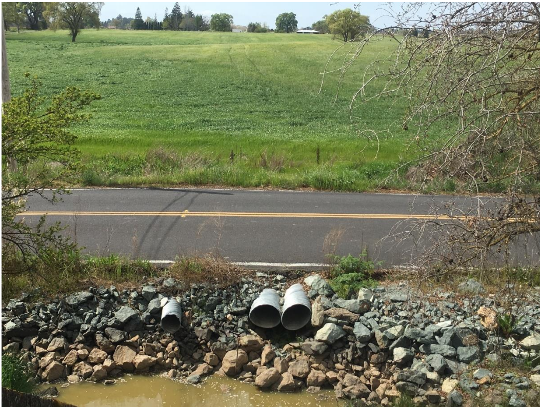
Photograph 2: UTR-R, looking west at the culverts for the proposed replacement.
