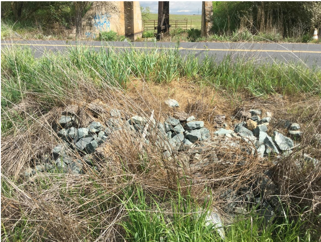
Looking east at downstream side of culvert into ditch
