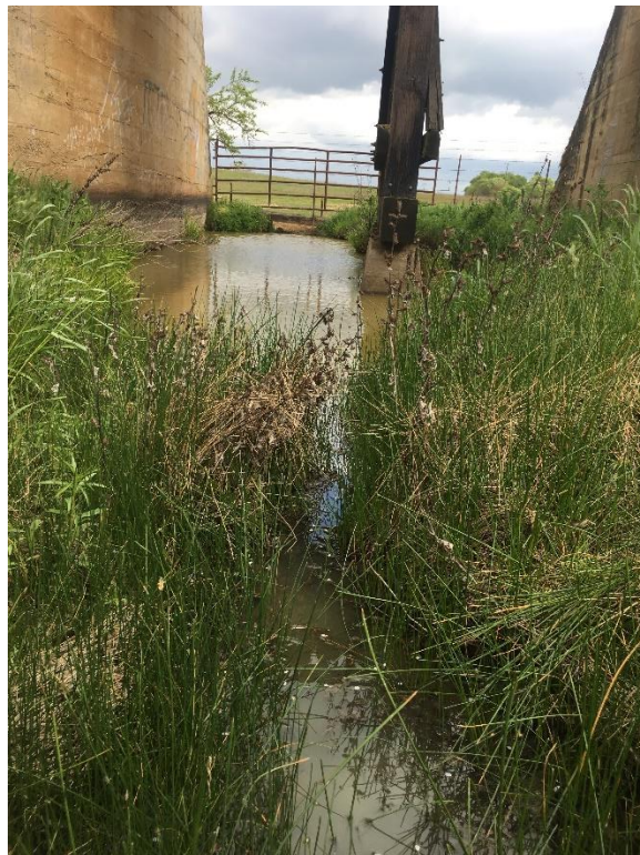
Photograph 6: Unnamed Drainage 1, looking down at the OHWM.
