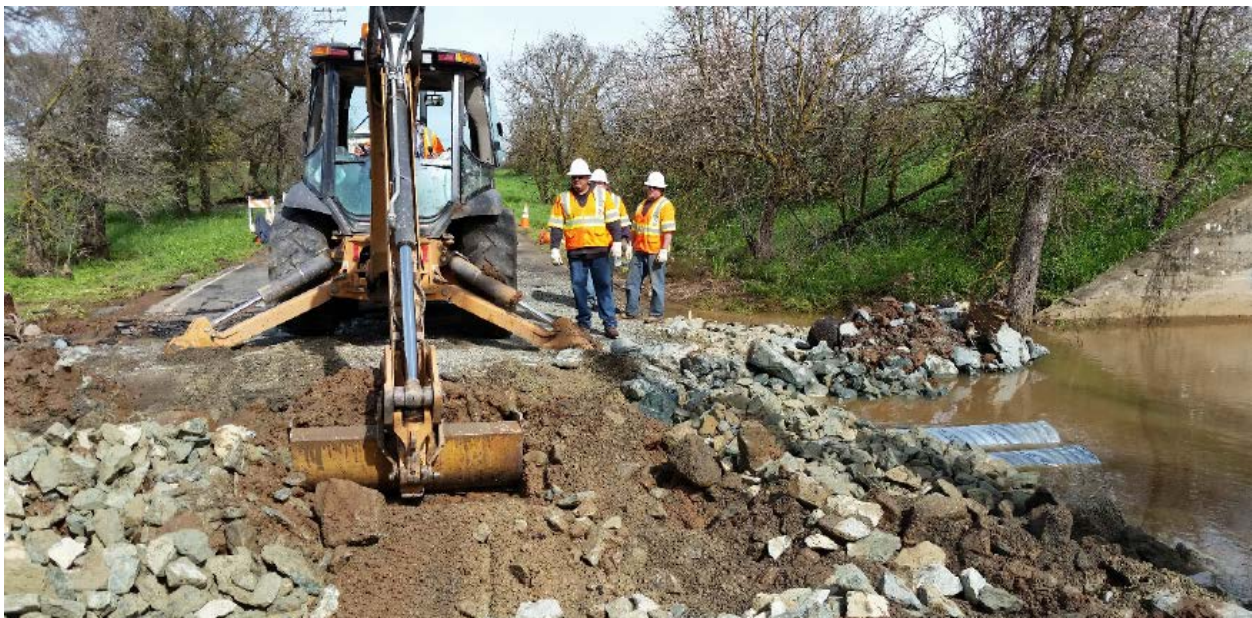
Figure 4. Emergency repair work - Railroad wing wall in right side of picture
