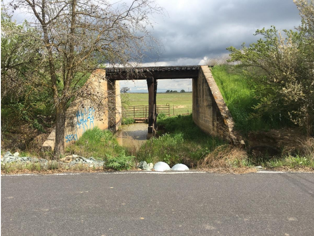
Looking east at railroad crossing
