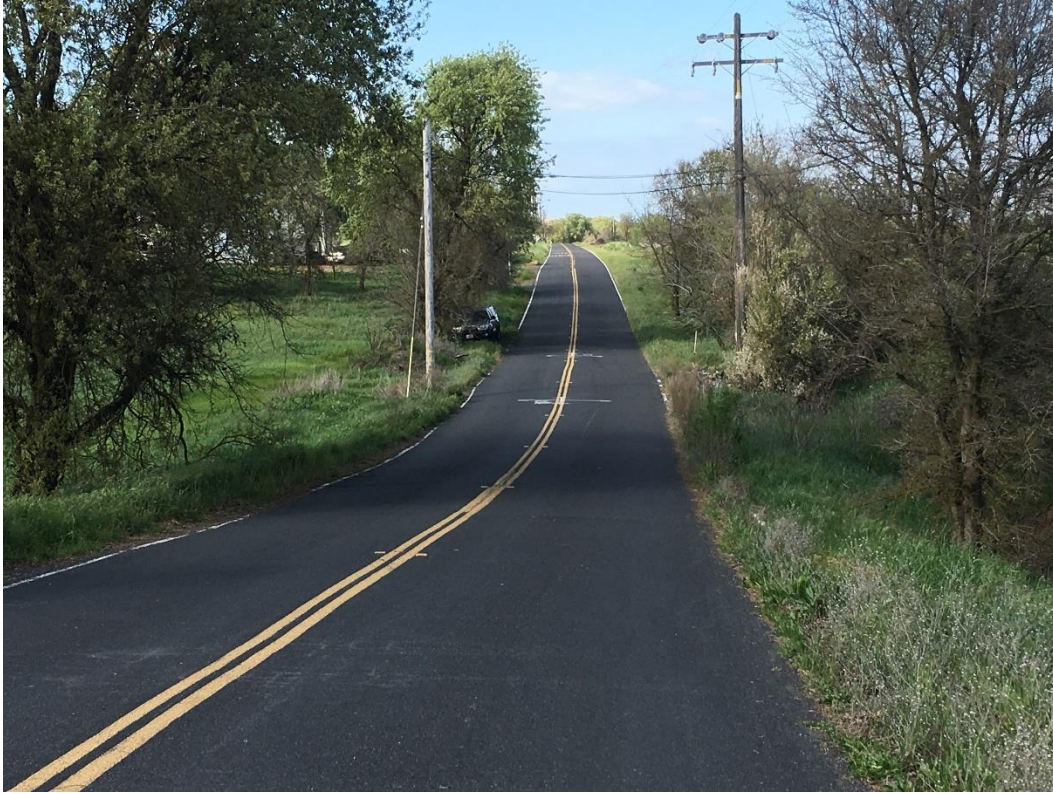
Photograph 1: Looking north toward culverts near the Liberty Road and Kennefick Road intersection.
