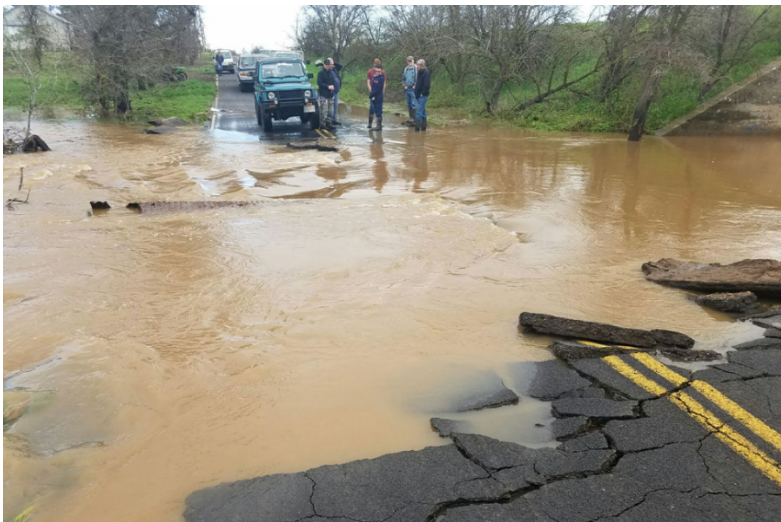
Exhibit 1 – Looking north on Kennefick Road
