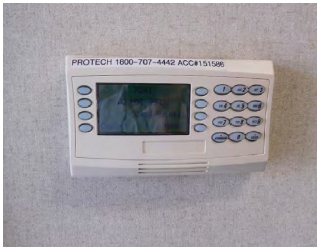
Figure 5 - Typical Alarm Keypad
