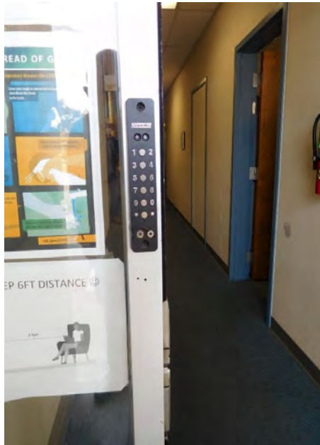
Figure 7 - Schlage KP78 Electronic Lock
