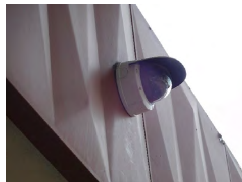
Figure 9 - Typical CDD Camera Installation
