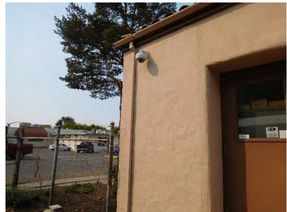
Figure 8 - Typical EHD Camera Installation
