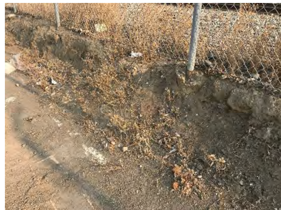
Figure 12 - Soil Undermining
