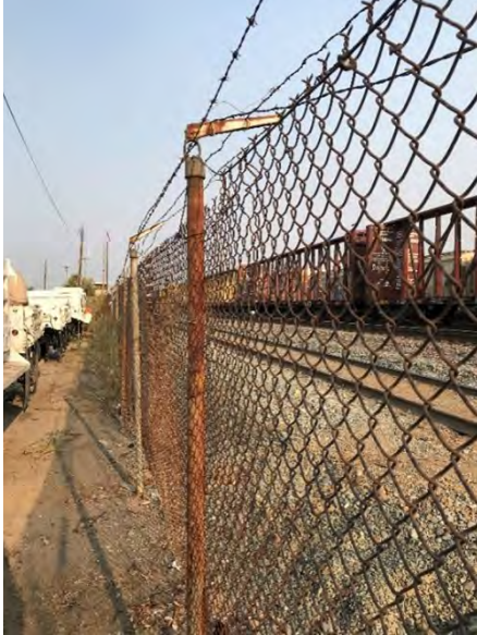
Figure 13 - The three-wire fencing topper is damaged and missing in some locations throughout the site
