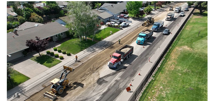
Water System Improvements in Colonial Heights and Lincoln Village
