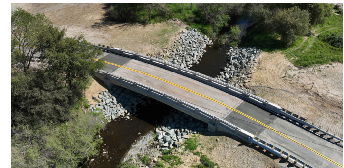
Bollea Road Bridge Replacement
