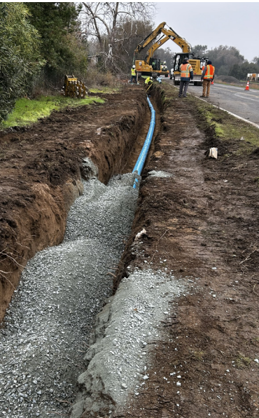
Thornton Water Main Installation
