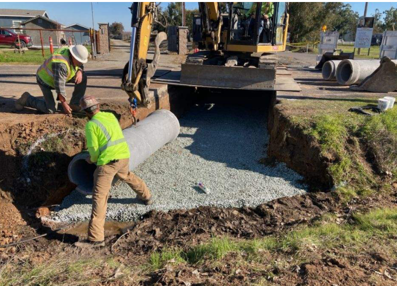
Fine Road Drainage Improvements
