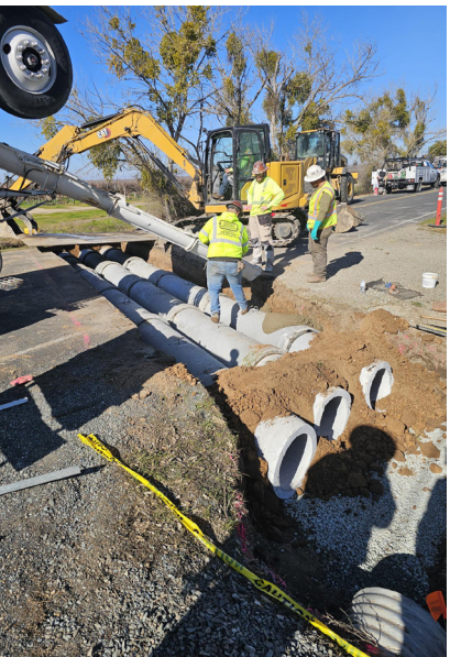
Fine Road Drainage Improvements
