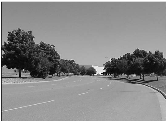
Existing Good Condition
