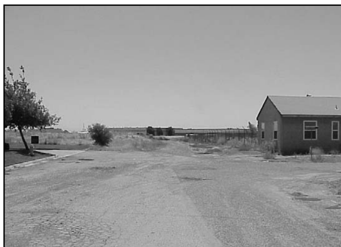
Existing Not So Good Condition
