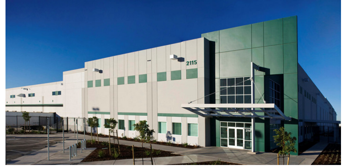
Figure 1.4.3 Unique architectural entrance canopy along with aggressive use of color provides strong building identity
