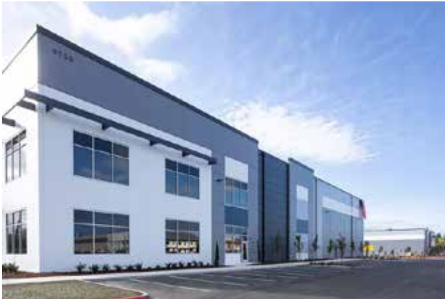
Buildings Should Generally be Concrete Tilt-Up
