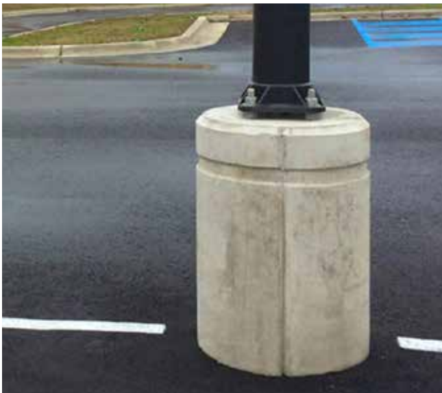
Design Light Pole Footings to Protect from Vehicular Damage
