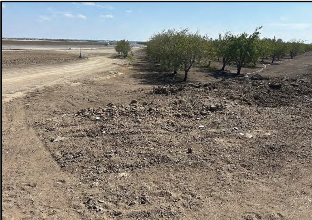
North edge of the north part of the site, looking east; 09/19/25. There is a newly constructed road adjacent to the north edge of the site.
