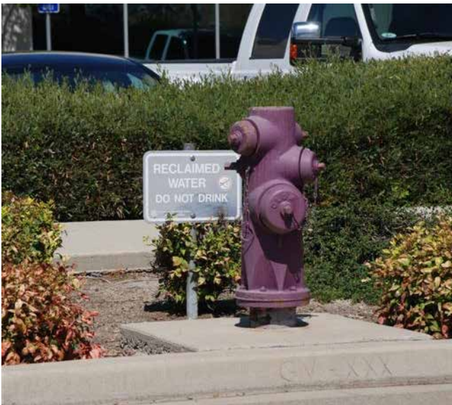
Reclaimed Water System
