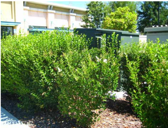
Exterior Utility Equipment Screened with Planting
