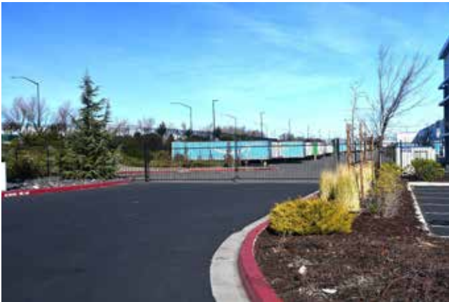
Match Security Gates to Fencing Design
