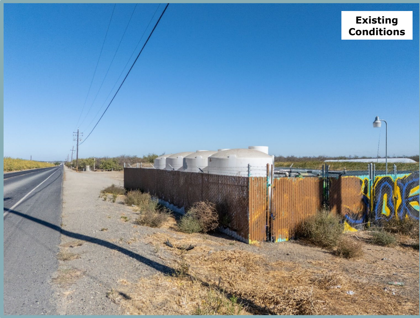
Figure 4.1-16 View 3: Existing Versus Post-Project Conditions South Chrisman Road Looking Northeast
