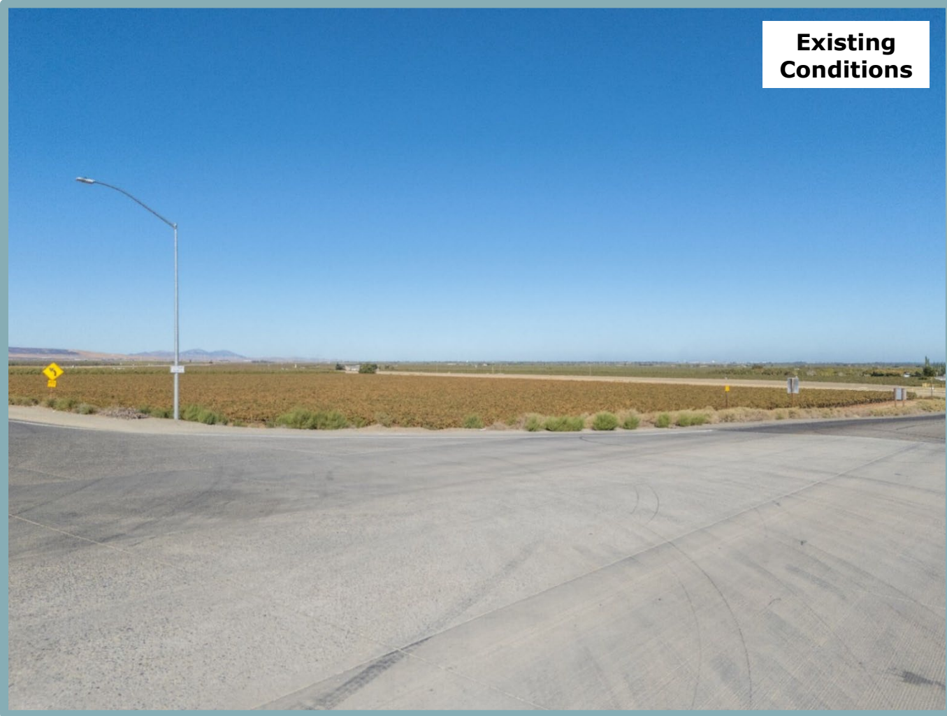
Figure 4.1-24 View 11: Existing Versus Post-Project Conditions from the Bird Road/SR 132 On-Ramp Looking West
