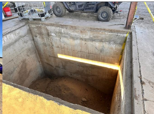
Photograph 114: View of Large Pit East of Main Shop Area.
