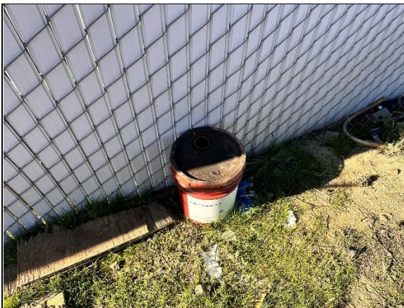
Photograph 85: View of 5-Gallon Pail Within Groundwater Supply Well Enclosure.
