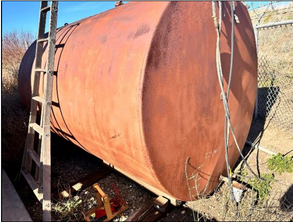
Photograph 69: View of Fuel Tank Servicing the Rigged Semi-Truck for the Well Pump.
