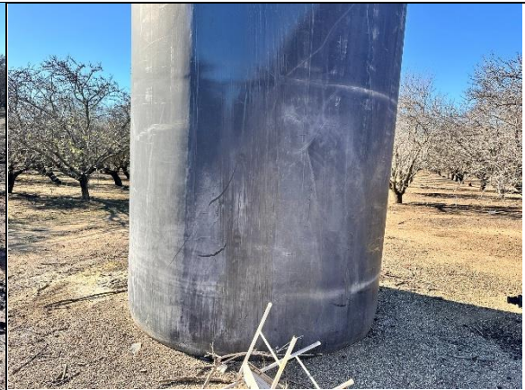
Photograph 76: View of Large Empty Tank Adjacent to Ash Mound.
