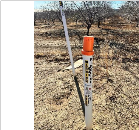
Photograph 37: View of Subsurface Pipeline Warning Marker Located in Central Area of Subject Property.
