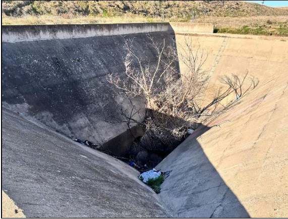
Photograph 47: View of Inside Pit Area.
