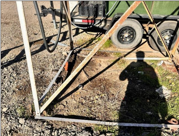
Photograph 111: View of Stained Area Beneath Fueling AST. Evidence of Strong Petroleum Odor As Well.
