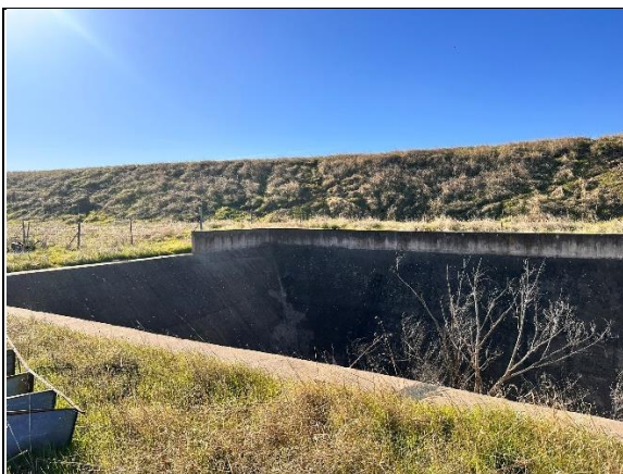
Photograph 45: View of Large Concrete Pit Adjacent to Aqueduct.
