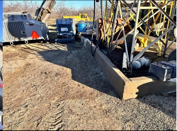
Photograph 2: View of Stained Soil Below Fueling ASTs. Strong Odors Observed Surrounding the Staining and ASTs.
