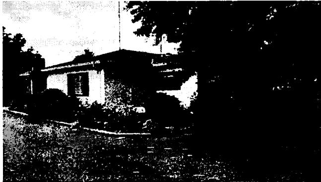
Photograph 4: Northeast corner of the residence. Camera facing southwest, September 9, 2025.
