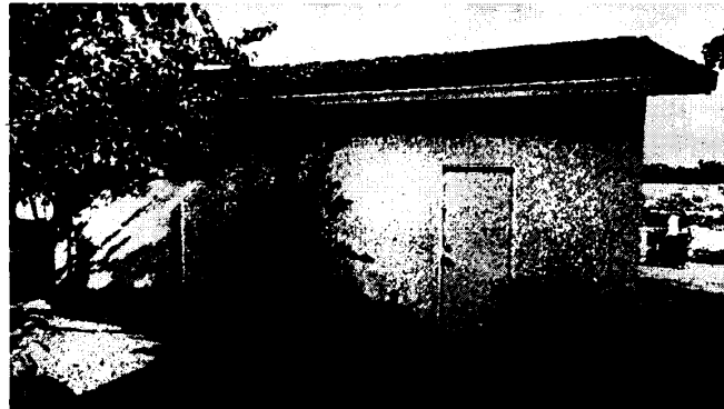
Photograph 8: South elevation of the garage, showing side entrance. Camera facing north, September 9, 2025.
