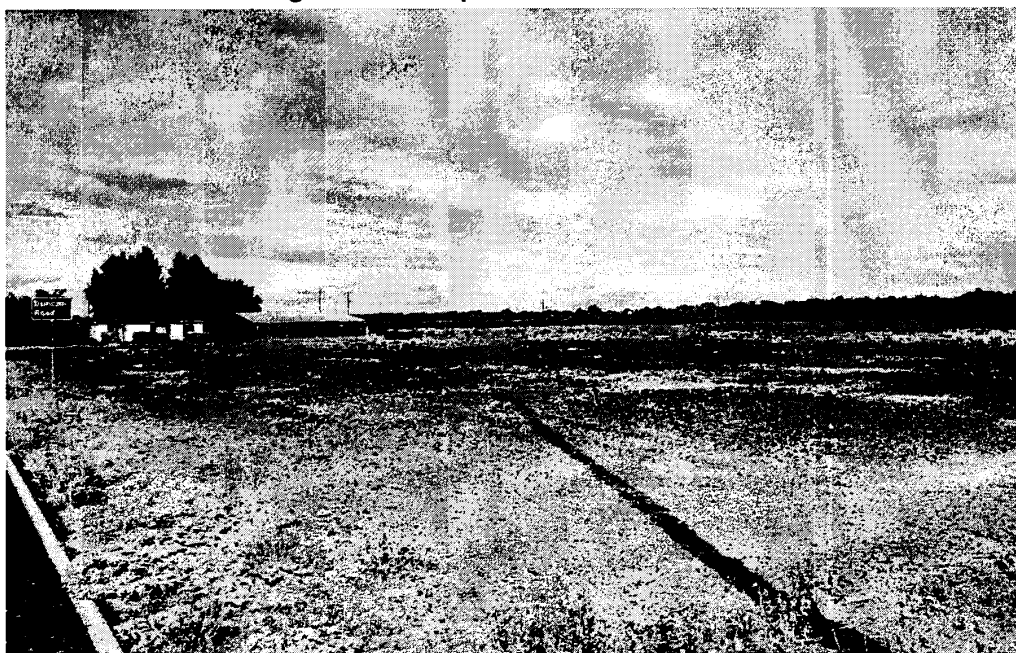
Figure 3 18133 East Comstock Road, showing the residence and barn at the left side of the frame. Camera facing northwest, September 9, 2025.
