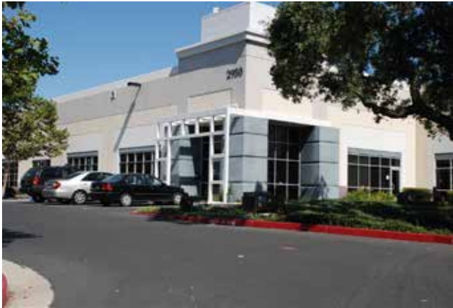
Utilize a High Window to Wall Ratio on Elevations Facing Vehicle Circulation
