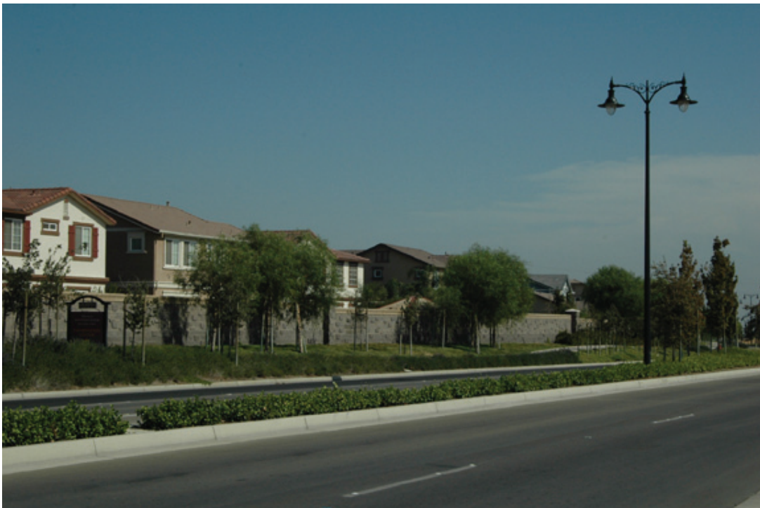
b. View along Mascot Boulevard, looking northeast, showing prototypical homes and streetscape within Neighborhood F.
