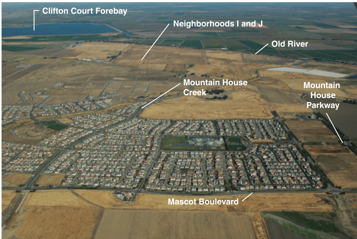
b. View looking north towards Old River and Clifton Court Forebay across recently-constructed Neighborhoods E, F, and G in foreground.
