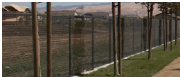
Chain Link Fence
