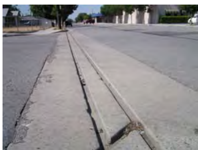
Bicycle unfriendly slot drain
