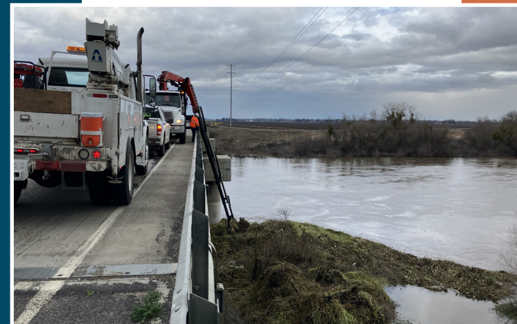
Airport Way Bridge Repair
