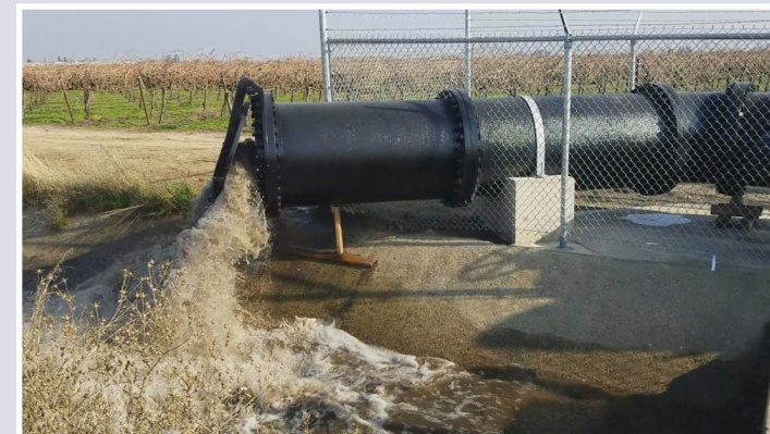
Acampo Area Flood Improvements
