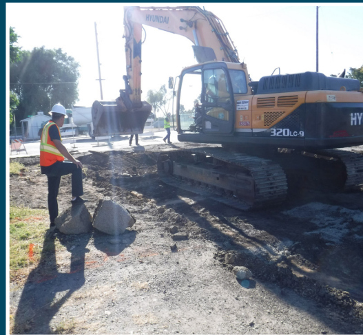
San Joaquin County Road Improvements
