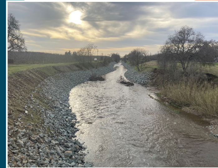
Mormon Slough Erosion Repair
