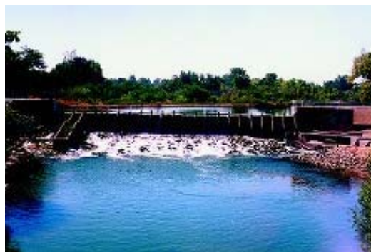
Woodbridge Dam diverts Mokelumne River water to Woodbridge Irrigation District.
