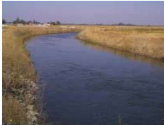
Lower Farmington Canal conveys Stanislaus River water to Central San Joaquin Water Conservation District and Stockton East Water District.
