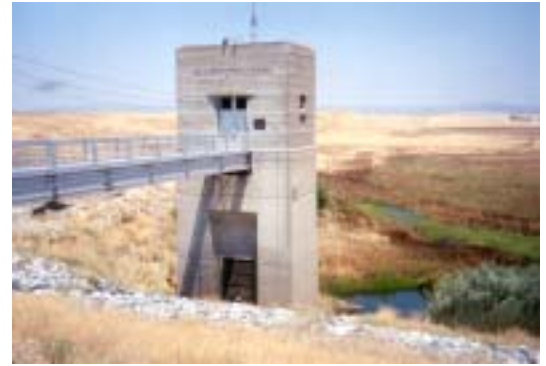
Farmington Dam provides flood control protection for areas downstream.
