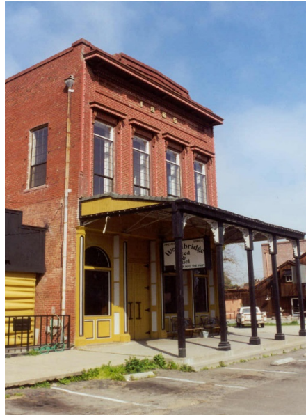
Bentley's General Merchandise and Wells Fargo Building
